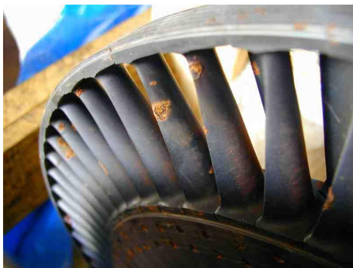
Figure 40 Turbine Blade Cracking
